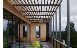
Gambar 3. Hamar Police Station Sumber:www.Archdaily.com, 2022
